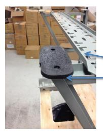
Attach the bottom brace use (4)  $1 \frac{1}{2}$ " X 3/8" bolt and (4) 3/8" washer. Place the washers from the top.
